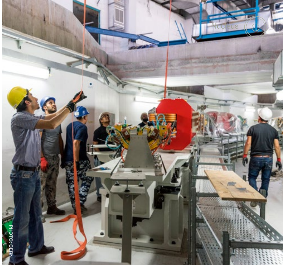
Workers inside the future SESAME building set up the synchrotron ring that now accelerates particles to nearly the speed of light
