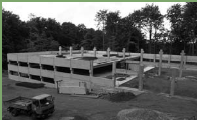
Step 4: Build some walls.
