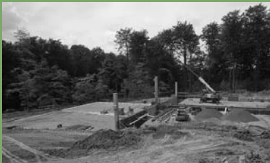
Step 2: Put down some foundations.
